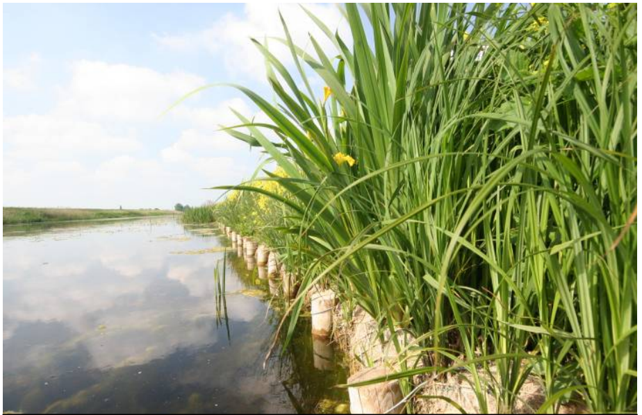
Sedges and other water plants growing in coir roll revetment on the Sixteen Foot Drain near Bedlam. Photo: Cliff Carson
