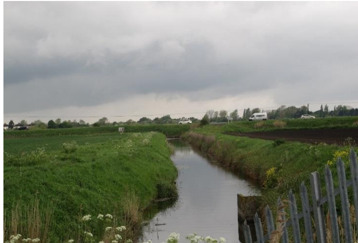
Western Spur Drain, Reach 7-8
