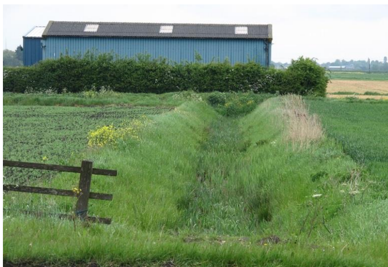
Southern Spur Drain, reach 29-30
