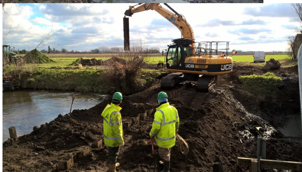
Refurbishment works on Marmont Priory Lock
