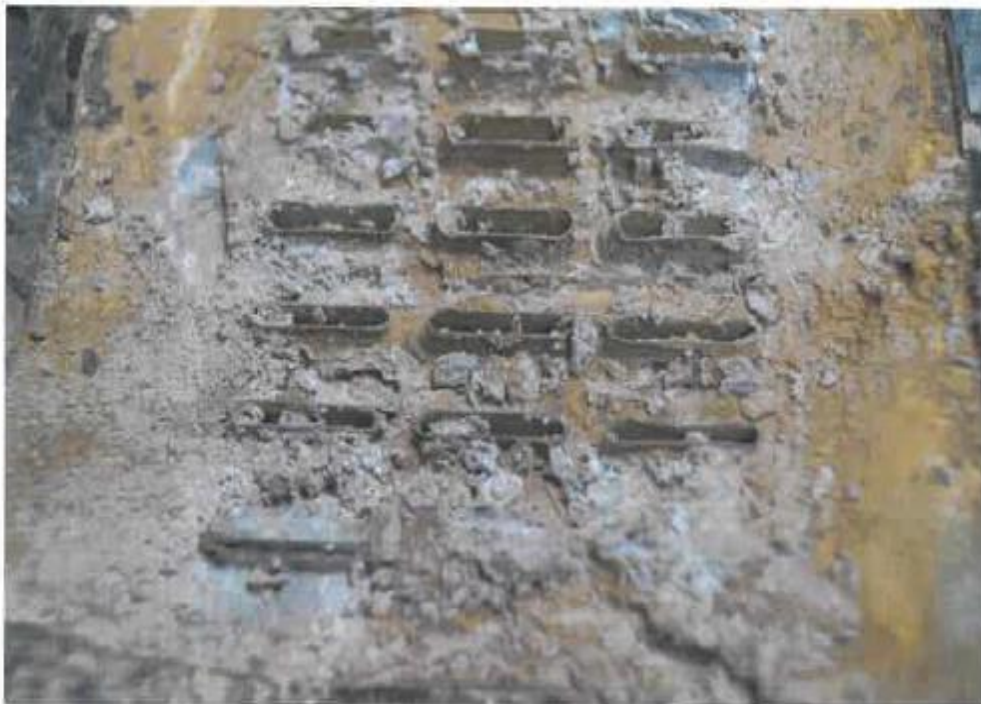
Figure 2. View of heat exchanger endplate "coolant side", showing copious deposits of corrosion product.
