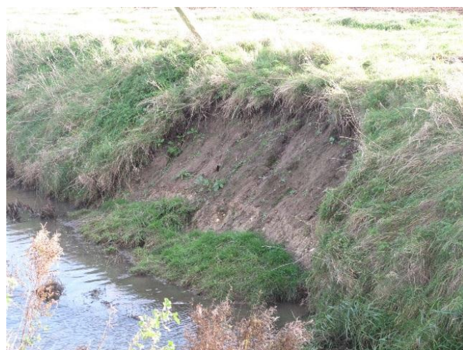
Bank subsidence, Latches Fen pumped drain, Reach 42-43
