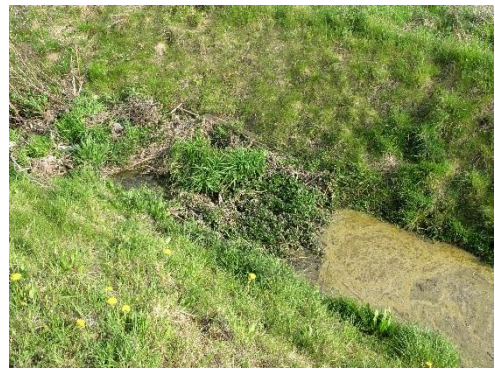
Bridge Lane Point 79
