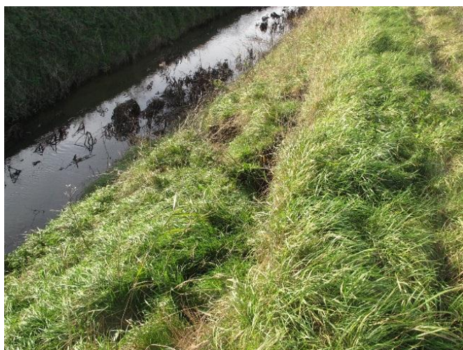
Bank subsidence, Latches Fen pumped drain, Reach 42-43
