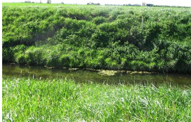
Reach 3-5 Binnimoor Road
