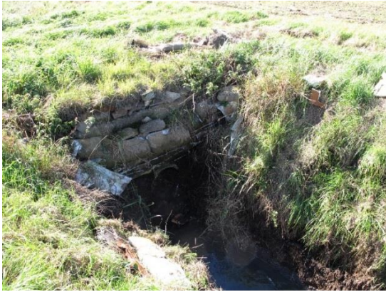
Failed culvert and collapsing headwall
