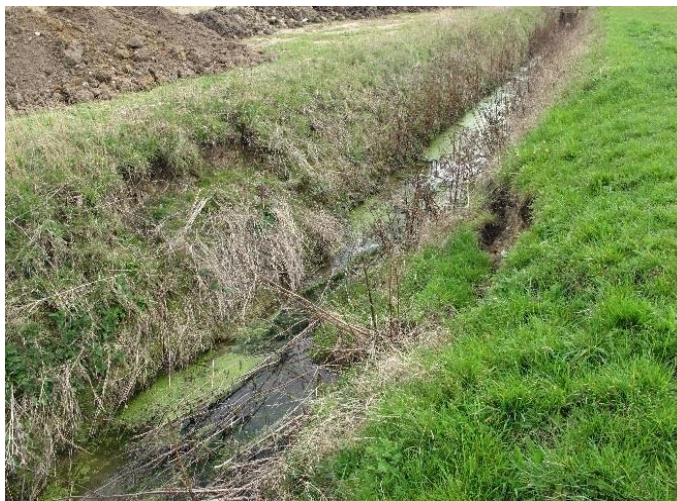
Bank Slips along reach 26-27
