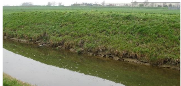
Bank slips along reach 2-9
