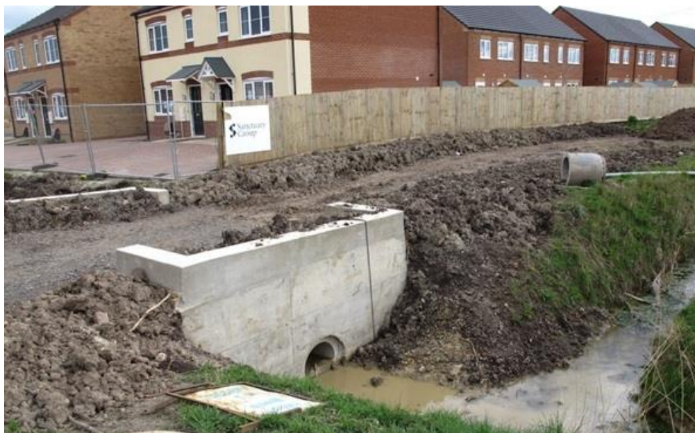
View of the access culvert from Gaul Road adjacent to Point 26 showing both the close boarded fence and deposited spoil within the Commissioners' maintenance access strip
