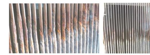
Should the pumps be required to pump in anger during a rainfall event and a build-up of weed occurs the screen is likely to collapse into the sump. It is recommended therefore that it should be replaced.
